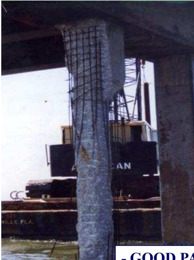
**- REMOVAL OF STANDARD JACKETS SHOWED THAT CONVENTIONAL ENCAPSULATIONS ALLOW CONTINUED CORROSION.**
