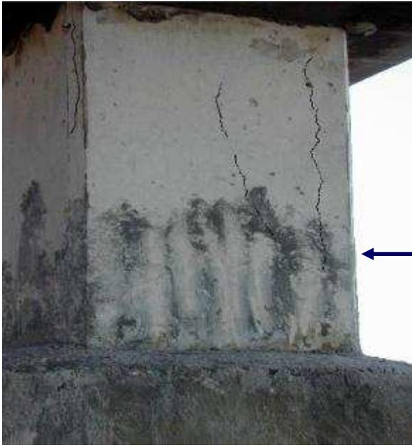
**- EVEN WHEN A GOOD ENCAPSULATION IS ACHIEVED, NEW CORROSION CELLS ARE DEVELOPED AND CORROSION CONTINUES**
