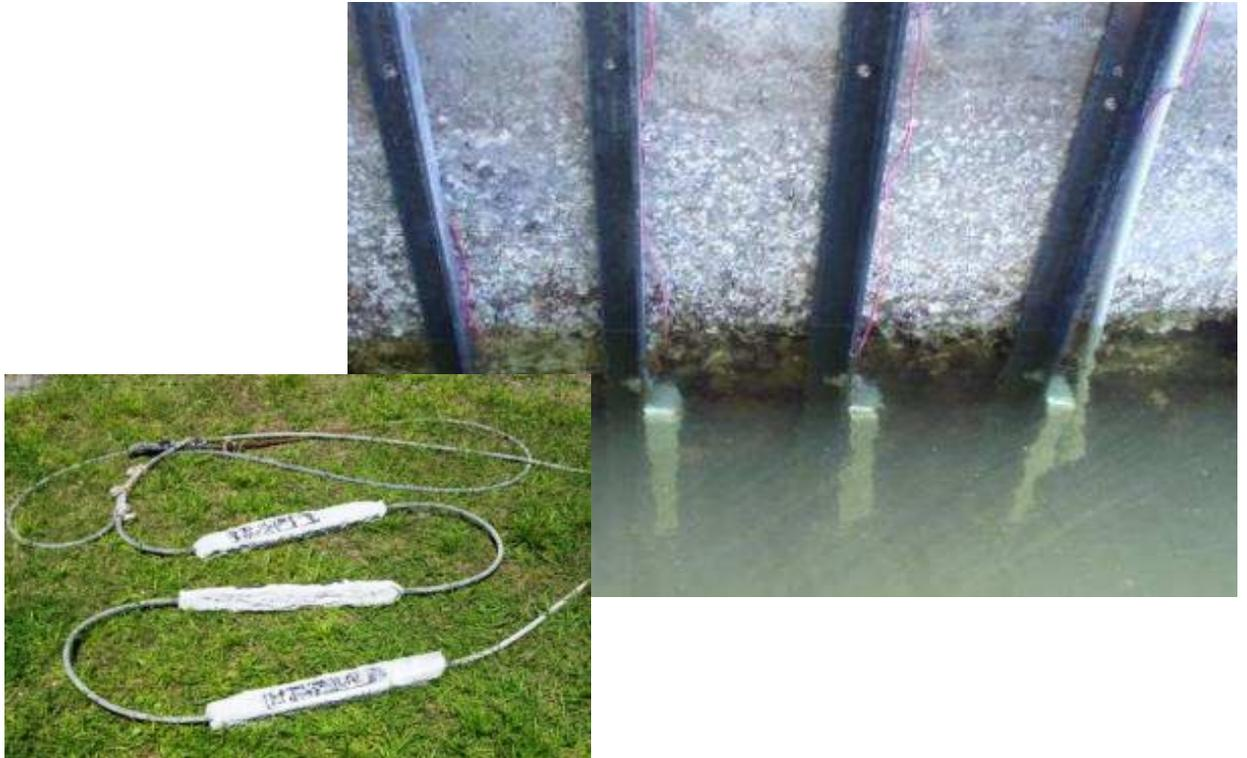
**THESE ANODES ARE MOSTLY USED TO PROVIDE CATHODIC PROTECTION TO STRUCTURES WITH UNDERWATER DAMAGE. SIMILAR ARE ALSO USED TO COMPLEMENT GALVANIC PILE JACKETS.**
